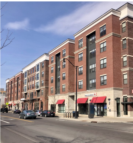
New Apartments North East Adjacent
